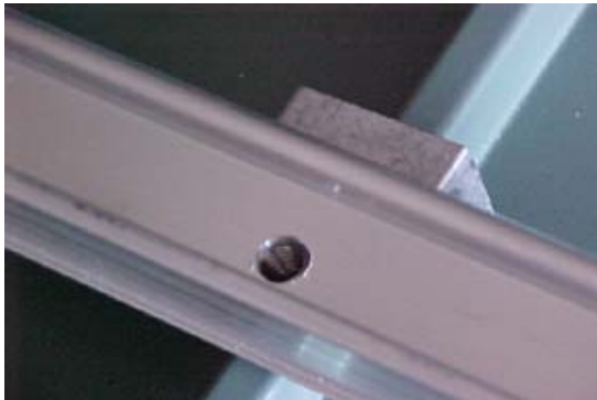
Hole Drilled in Channel
