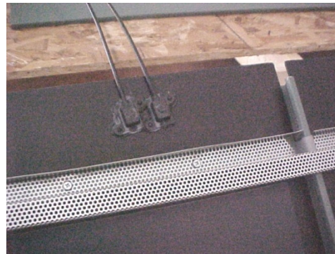
Installed Z-Closure, ready for quick connection
