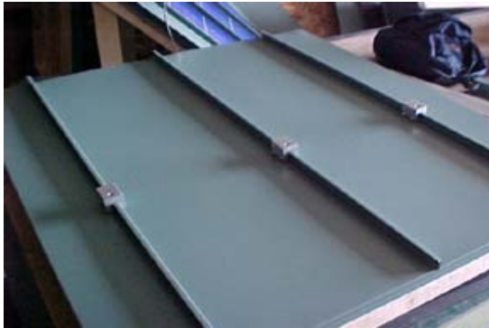
Mounting Blocks Installed
