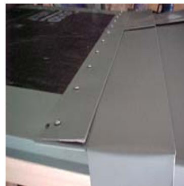
Installation of Starter Cleat
