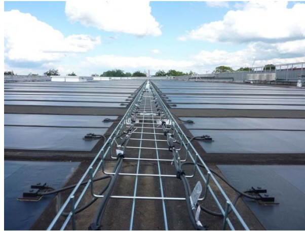
Figure 31: Uncovered Wire Mesh Cable Tray – Installation in Progress
