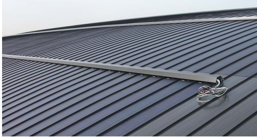
Figure 33: Custom Wireway Installation Matching Existing Metal Roof
