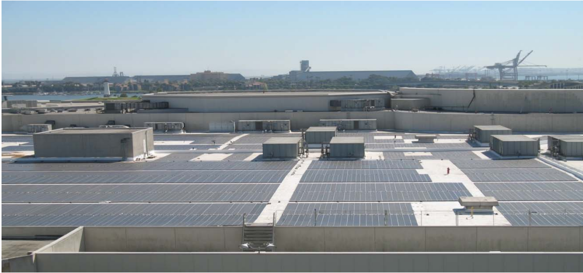
Figure 4: Reference Project Photo for Direct Bond to Single-Ply Membrane Roofs
