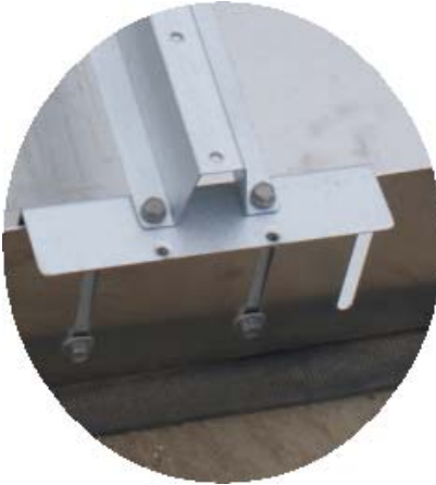
Figure 40 Support Rail secured to risers of Base Support
