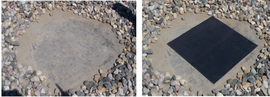
Figure 37 Base Support- Roof Preparation
