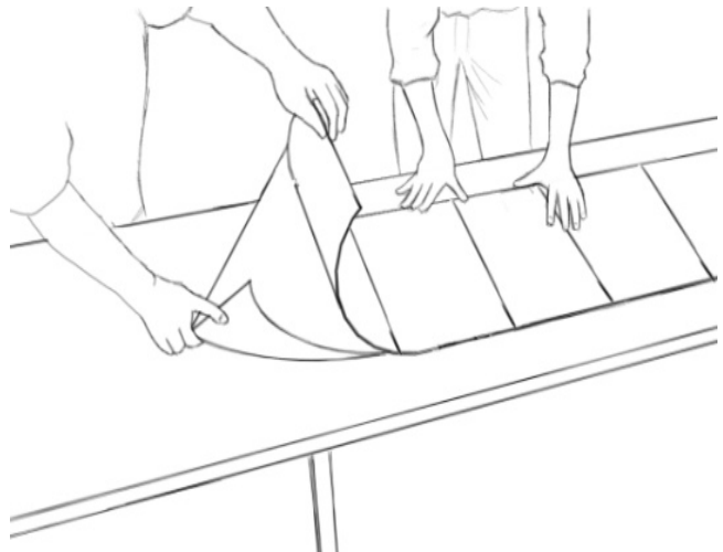
Figure 6 Installation of PVL
