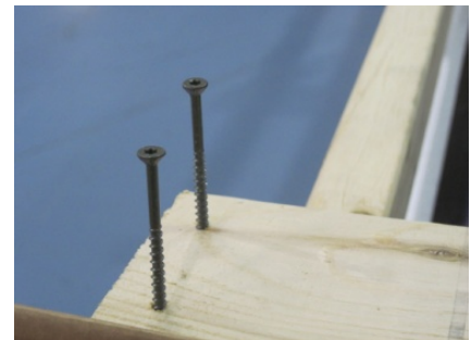
Figure 29 Screws Securing Cross Braces
