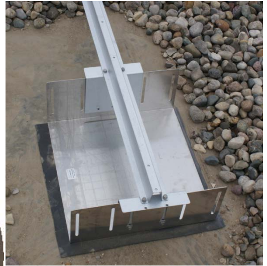
Figure 40 Support Rail secured to risers of Base Support
