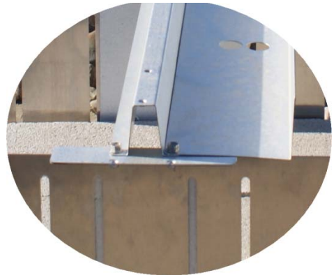
Figure 40 Support Rail secured to risers of Base Support
