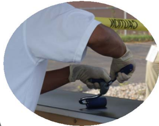
Figure 9 Use J-Roller to press out air bubbles
