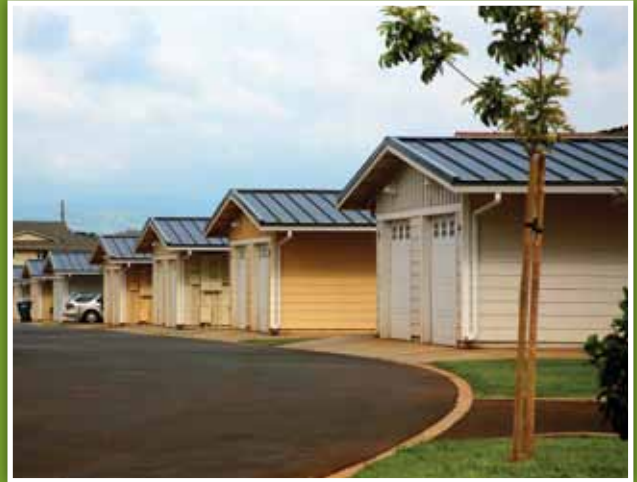
U.S. Army Installation | Oahu, HI | 6MW
