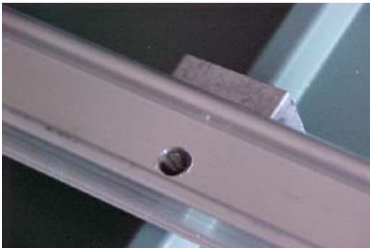
Hole Drilled in Channel
