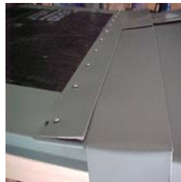
Installation of Starter Cleat
