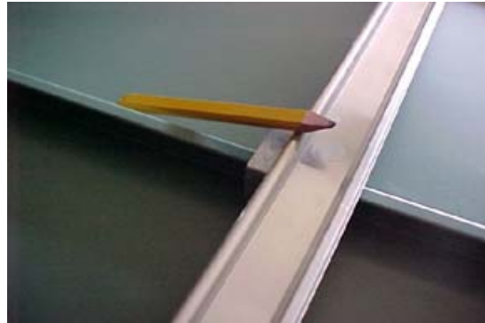
Snow Guard Channel in Place
