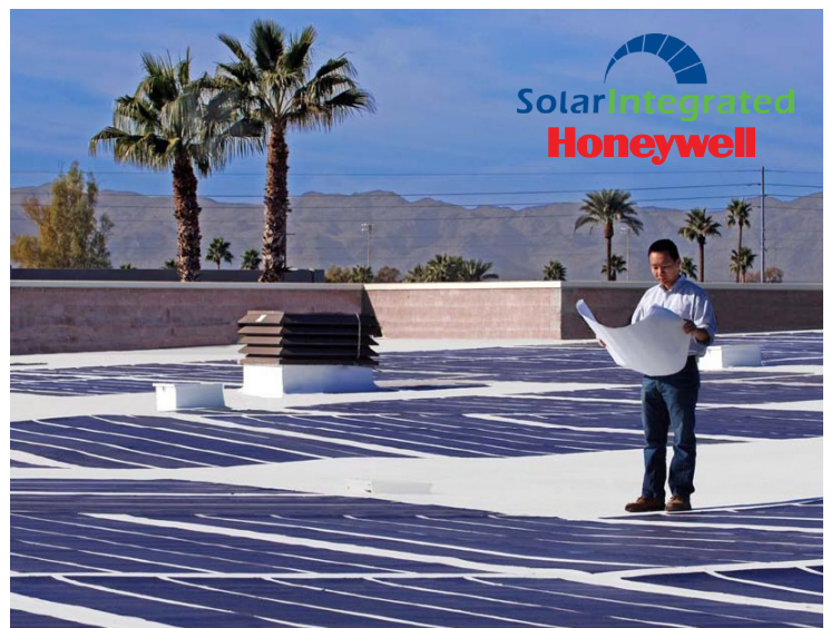
Luke Air Force Base (375 kW) Glendale, Arizona
